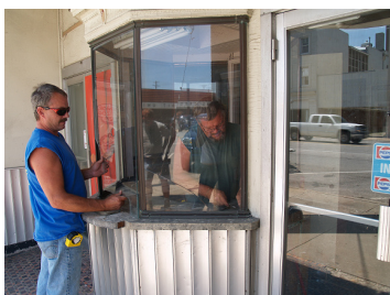
Glass Depot replacing the ticket booth glass
